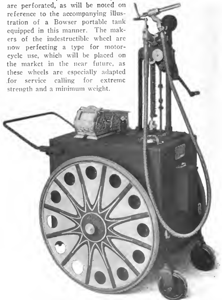
Bowser Garage Tank with Indestructible Steel Wheels.
